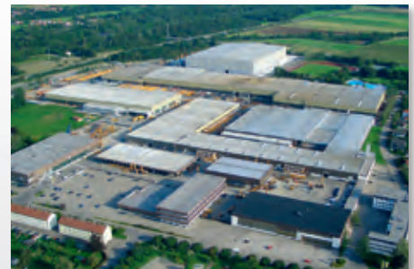
Kirchdorf: hydraulic cylinders
