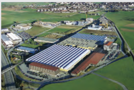
Bulle: diesel engines, splitter boxes, hydraulics
